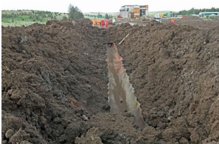
Figure 1: Result of a Full-Scale Test to Verify Fracture Propagation Arrest Capabilities for a Dense-Phase CO 2 Pipeline
