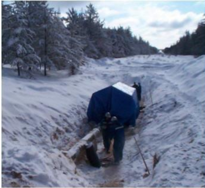
Figure B.6: Hording-In an Excavation Site for Winter Recoating.
