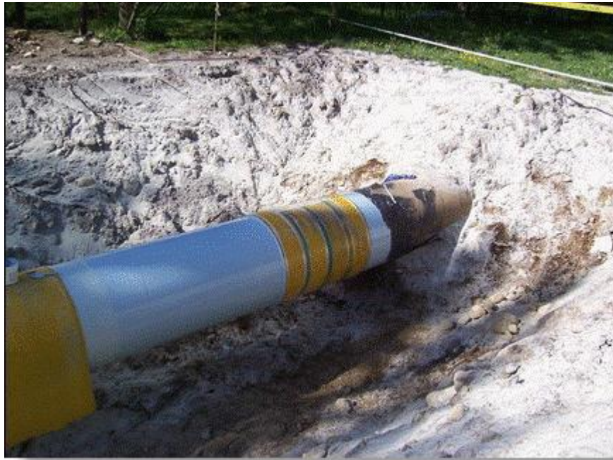
Figure E.14: Composite Reinforcement Sleeve Repair.
