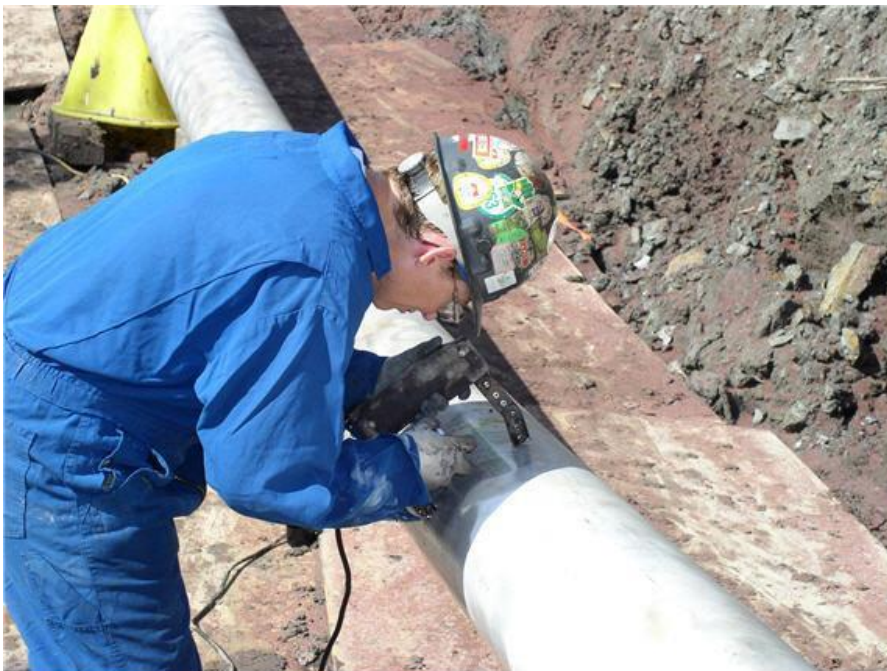
Figure B.2: Top of Pipe In-the Ditch SCC Assessment Using BWMPI.
