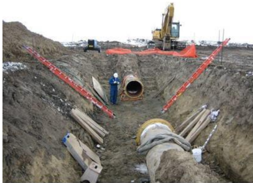
Figure E.15: Repair by Pipe Replacement.
