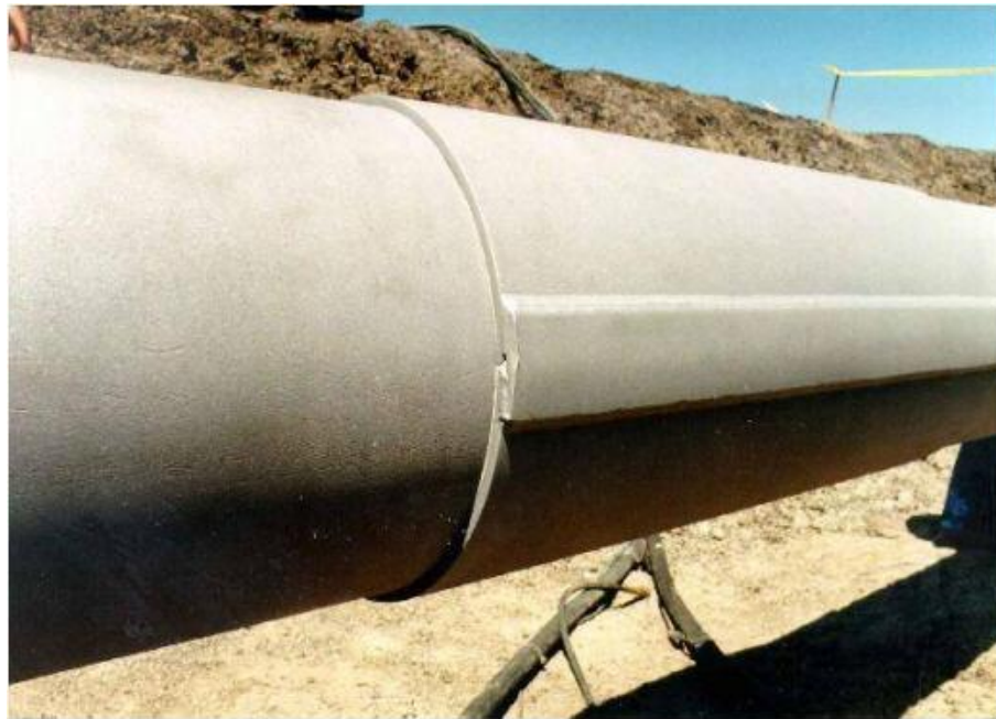
Figure E.12: Steel Reinforcement Sleeve.
