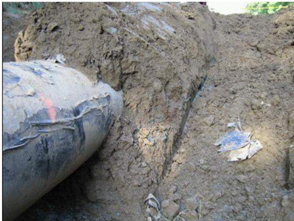
Figure 2.2: Polyethylene Tape Coating Showing Evidence of Disbondment.
