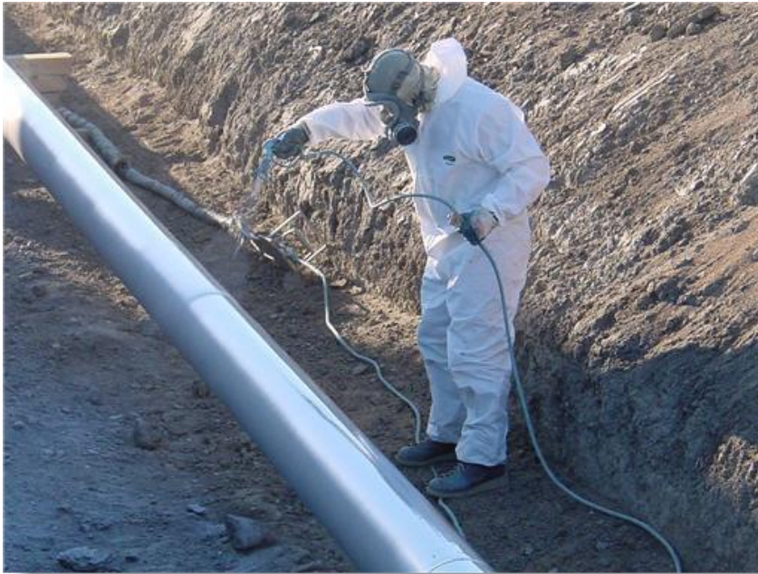
Figure B.5: Application of Liquid Based Coating after Bell Hole Inspection.
