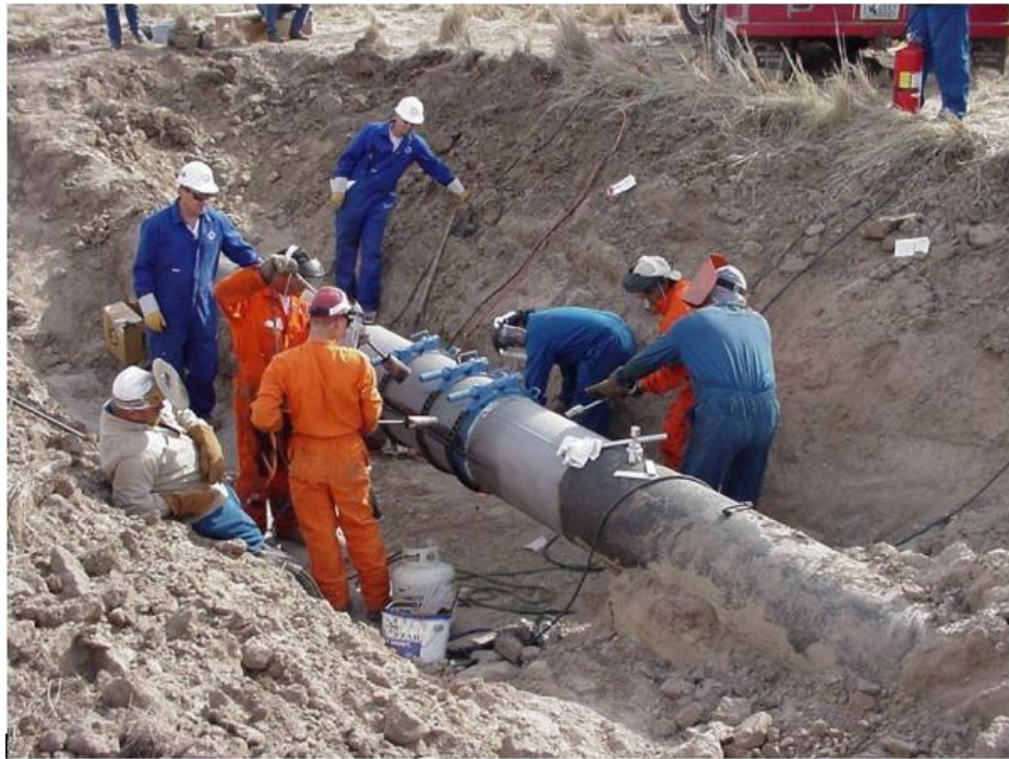
Figure E.13: Installation of a Reinforcement Sleeve After SCC Removal.
